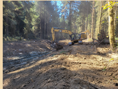
Whole trees being added to the excavated backwater portion of the project.
