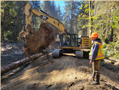
Whole trees being added to the excavated backwater portion of the project.
